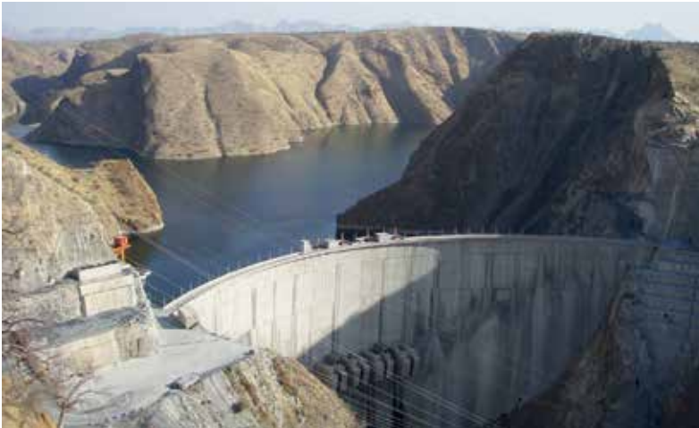
Above: Tekeze Hydropower Project
