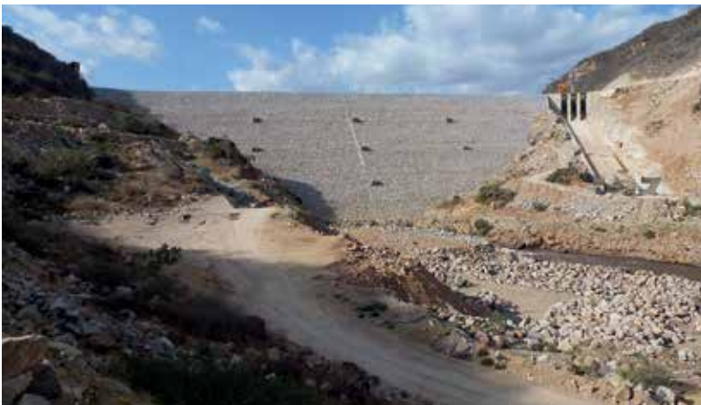
Above: The Genale Dawa III Hydropower Project
