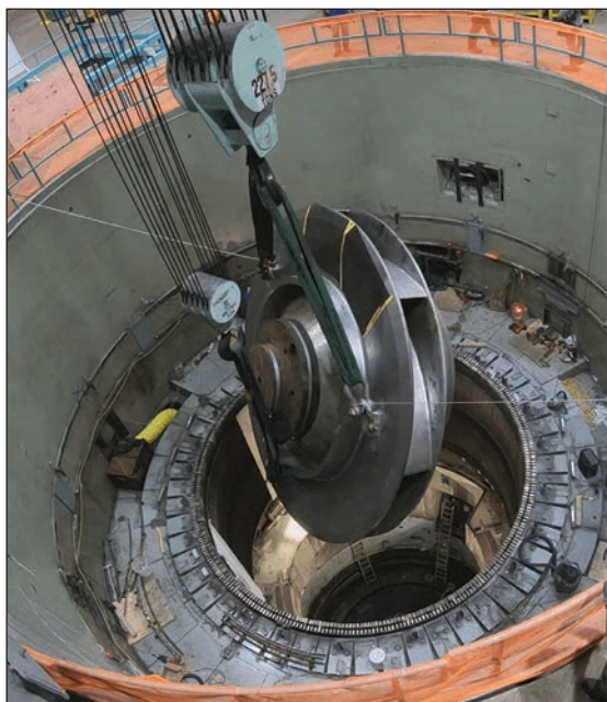
Removal of the original pump-turbine runner from Unit 2 at Bad Creek.
