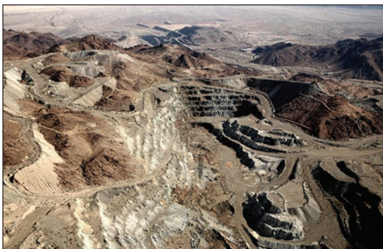
The Eagle Mountain pumped storage project, which will be an integral component of California's renewable energy policies, and its goals for reduction of greenhouse gas emissions.
